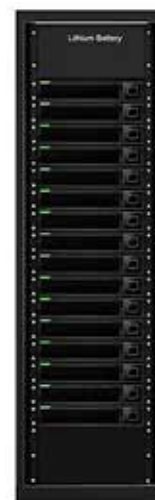
96kWh Lithium Battery
