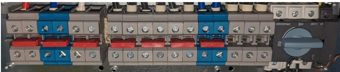
Figure 3.3a 10-20KVA CABLE CONNECTIONS
