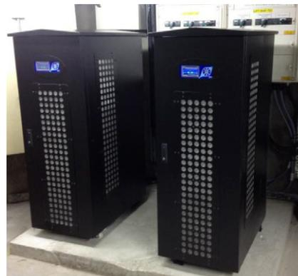
2x 80kVA High Internal Protection IP42 UPS supporting residential lifts in the UK
