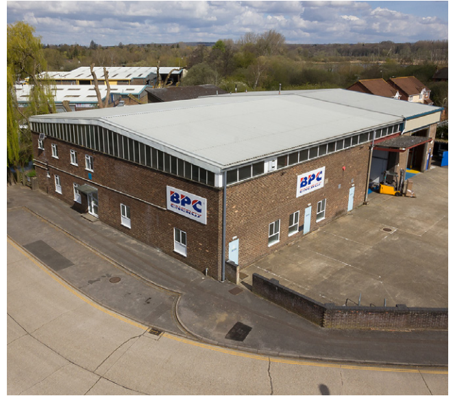
UK Romsey manufacturing operation
