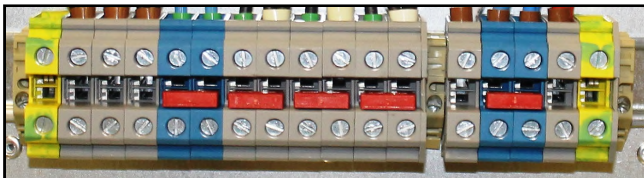
Figure 2.2 10-15-20-30 kVA Cable Connection
